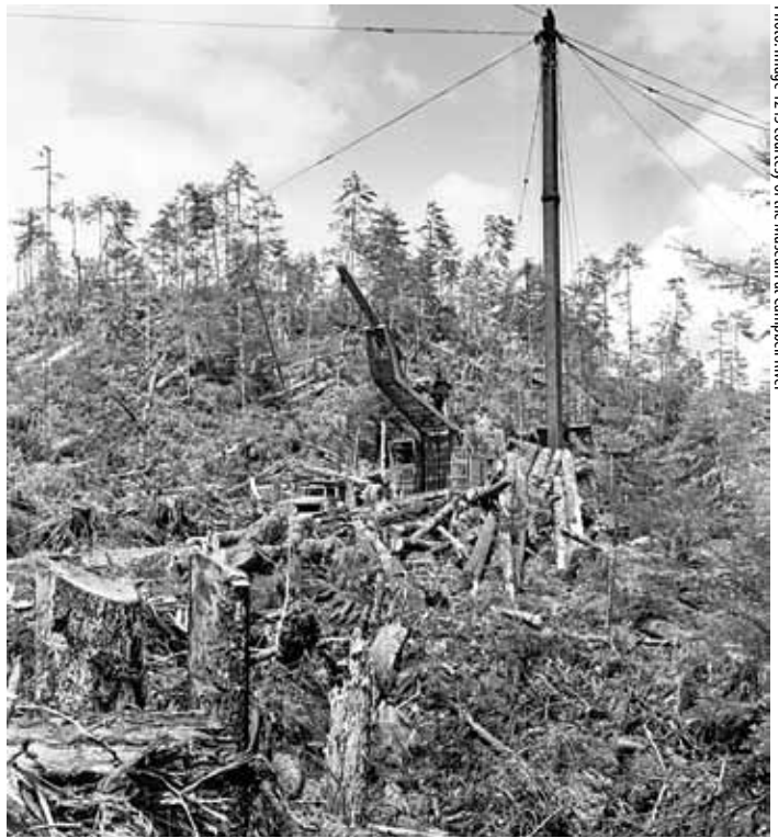
Taken in 1968, this photo shows a slightly more modern steel spar and a heel boom loader.
