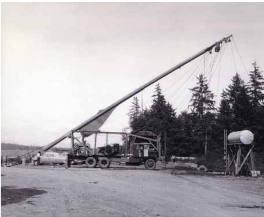
The first prototype “Madill Mobile Spartree” arrives at Baikie Bros. Logging in 1956. It’s mounted on an ex-military rubber-tired carrier provided by Baikie Bros.
