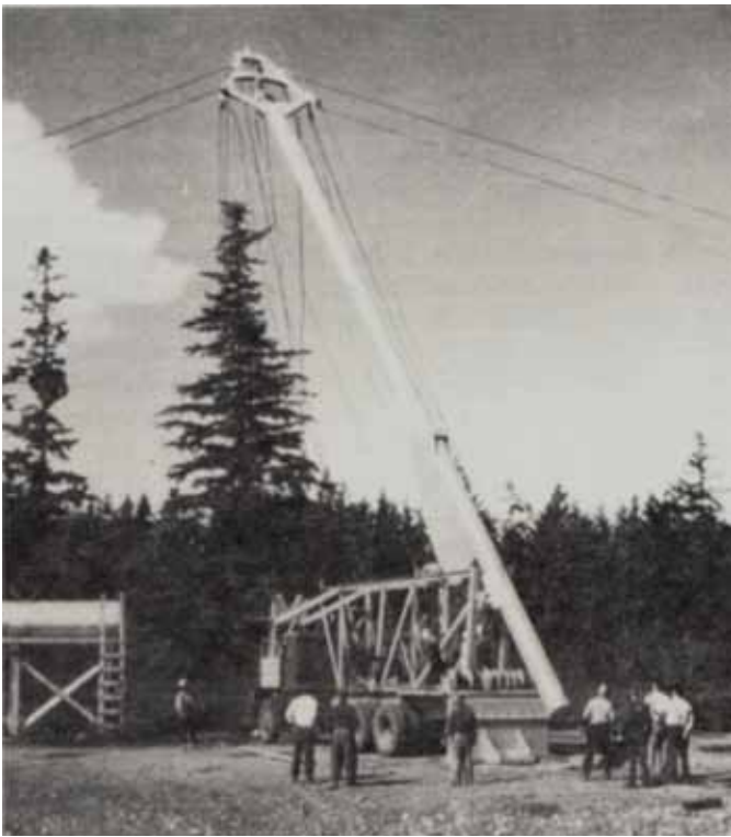
Demonstrating how the tower is erected on Baikie Bros. land near the present day Freshwater Marina.
